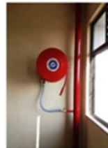
INTERNAL HYDRANT & HOSE REEL
