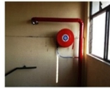
INTERNAL HYDRANT & HOSE REEL
