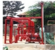
PUMP ROOM WITH AIR VESSEL TANK ARRANGEMENT
