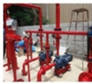
ELECTRICAL, DIESEL & JOCKEY PUMPS
